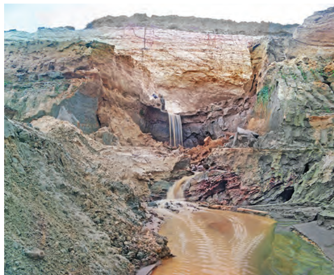
Here ground-water within the Folkestone Sand, held up by a seam of car-stone, is seen surfacing, eroding a small canyon
